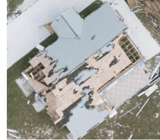
Structural roof damage
