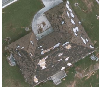
All layers roof damage
